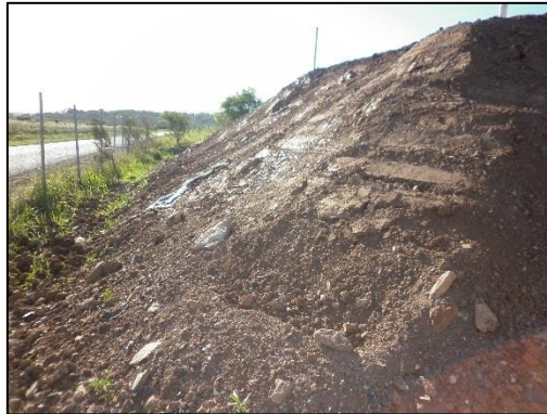
Figure 5. Photo of site.
