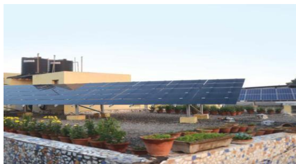
Figure. 5: Integration of green roof and RiPV system
