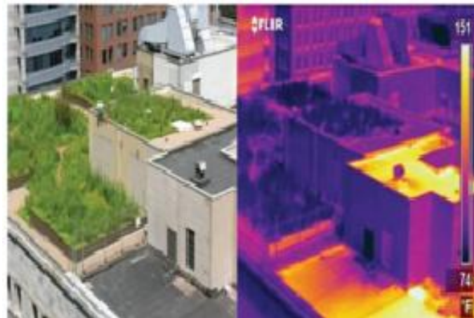
Figure 6. Thermal mapping of rooftop with greeneries & black coating
