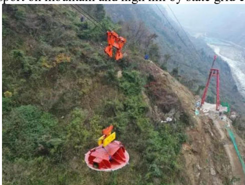
Figure 2. 15-ton mountain freight ropeway lifting 9.8-ton spools
